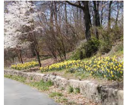
The stone wall is one of the most distinct features but is in poor repair.
