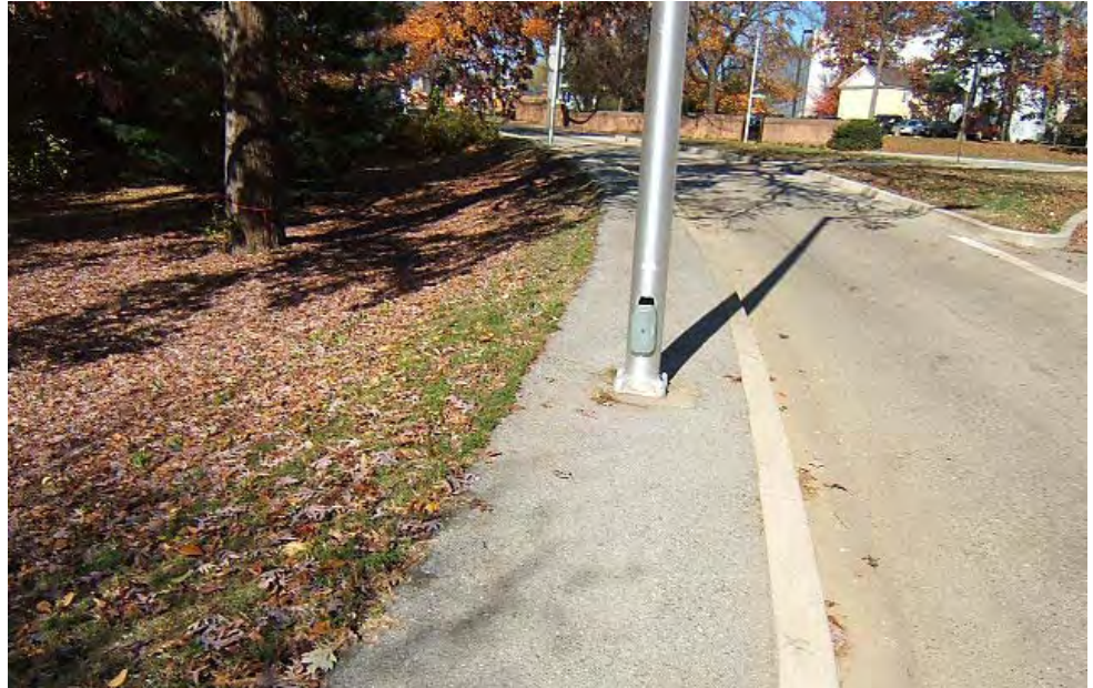
Existing sidewalk along busy roadway is narrow and obstructions inhibit ADA access.
