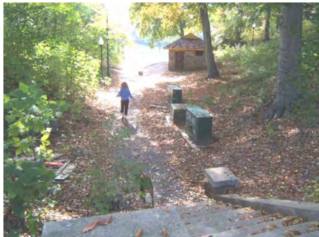
Low wall and overgrowth block most important vista of Lower Lawn (top left). Steps are uninviting and do not provide ADA access (top right). Presence of transformers and old restroom structure along with overgrown vegetation create uncomfortable environment, particularly for the main entrance to the Dell (left).
