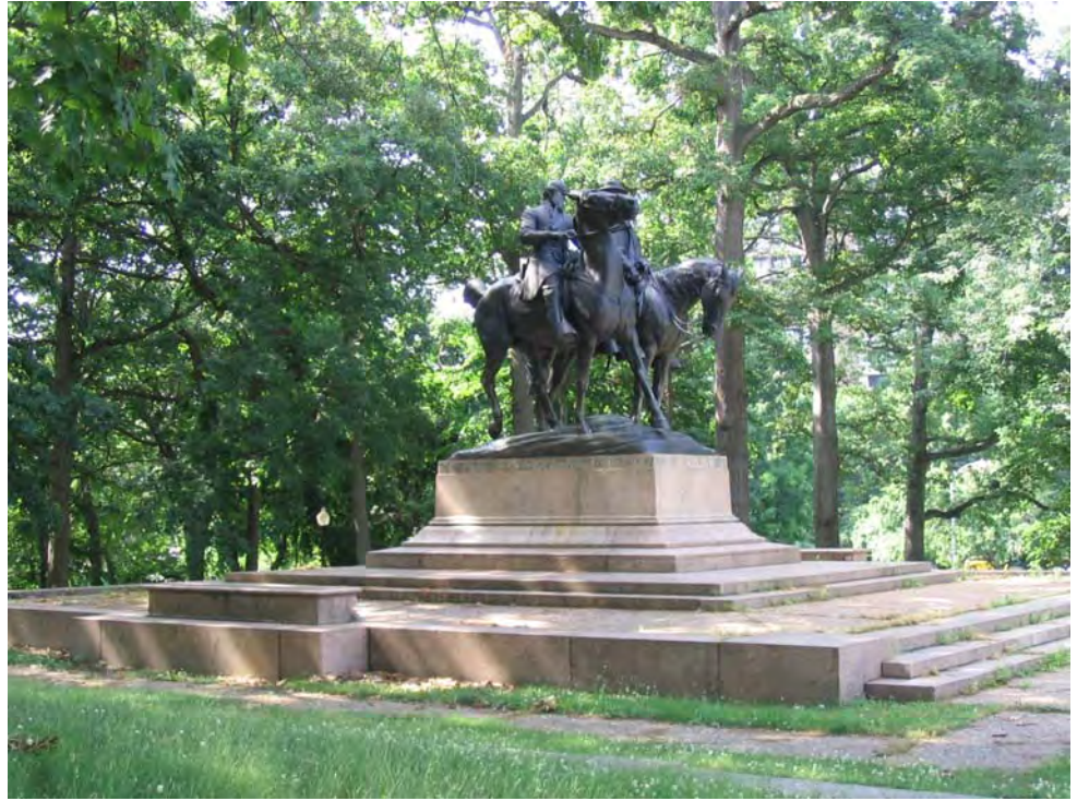
The lower plinth to the Lee and Jackson Monument is not ADA accessible, nor is interpretation provided.
